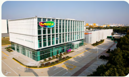
Life Science Wuxi Office Building
